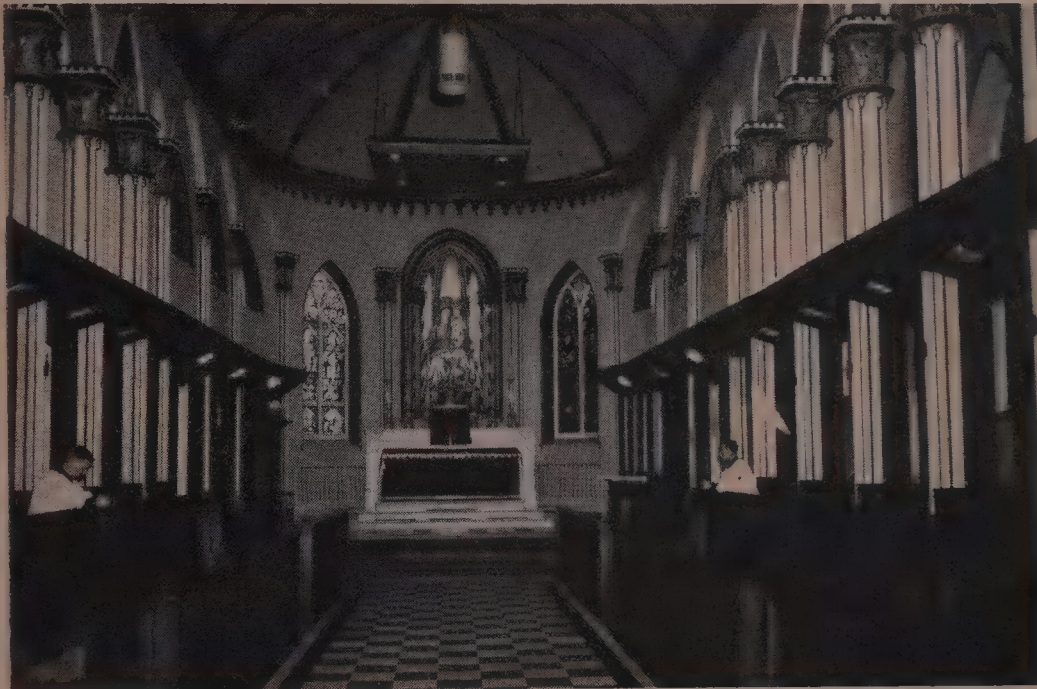
Recently renovated chapel at Paca St.
